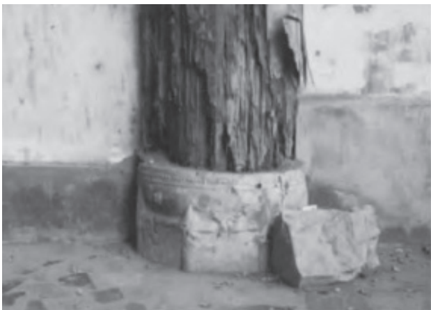
>图2 柱根腐朽
