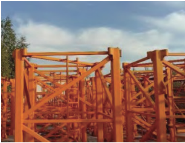
> 图3塔吊安装前构件检测
