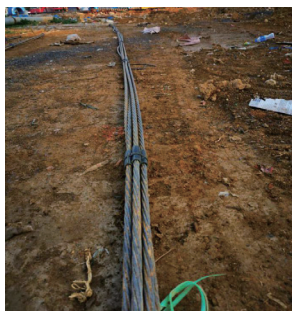
> 图6 复合锚杆杆筋制安 > Fig.6 Fabrication and installation rebar of composite anchor
