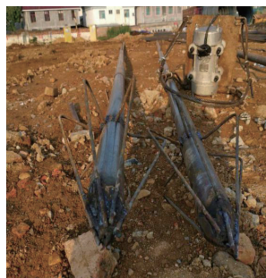
> 图5 复合锚杆杆骨制安 > Fig.5 Fabrication and installation bone of composite anchor
